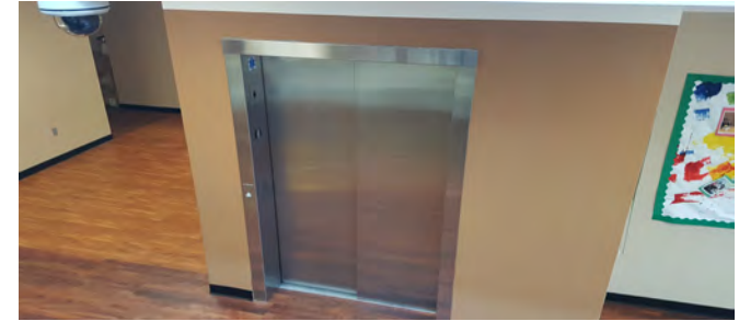
9 Passenger Elevator & Freight Service for Lower Level
