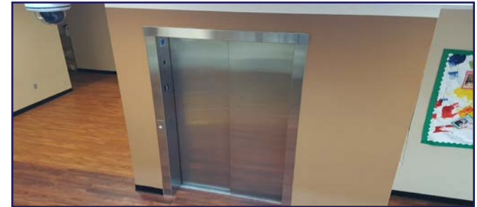
9 Passenger Elevator & Freight Service for Lower Level
